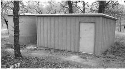
Storage Building and water tank
